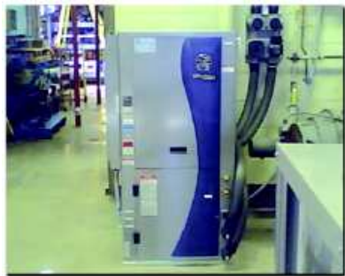
This WaterFurnace® flow center and Envision® machine is used for heating the lab featuring the worlds first 30 EER (cooling efficiency) and 5 COP (heating efficiency) comfort system.
