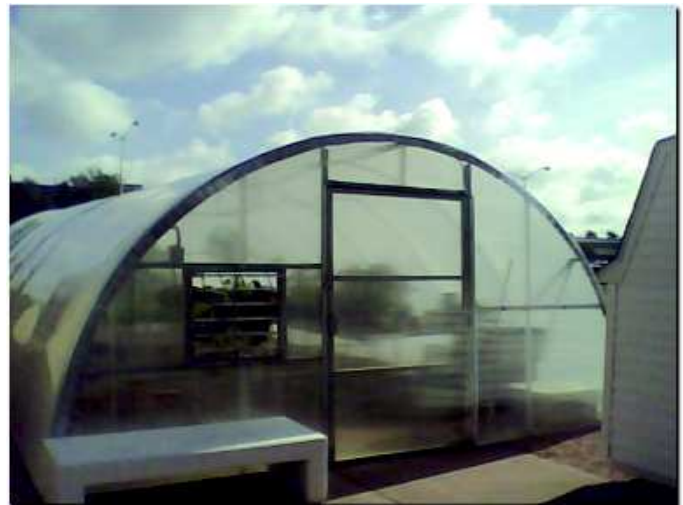
CVTC Greenhouse has replaced fossil fuel heating with geothermal heating.
